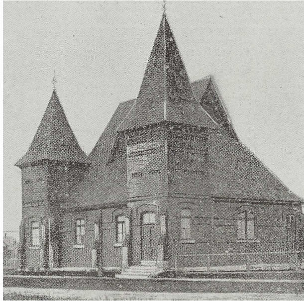
Historical photograph of Annette Street Baptist Church, prior to 1906 when the building was extended to the west and altered (Source: The Leader and Recorder (Winter 1996), 8)
