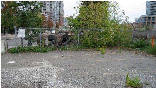
Plate 3: Looking east at parking lot, location of proposed Douro Street bridge landing
